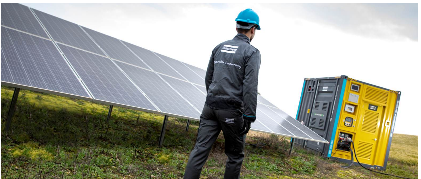
Solar panels not included.
